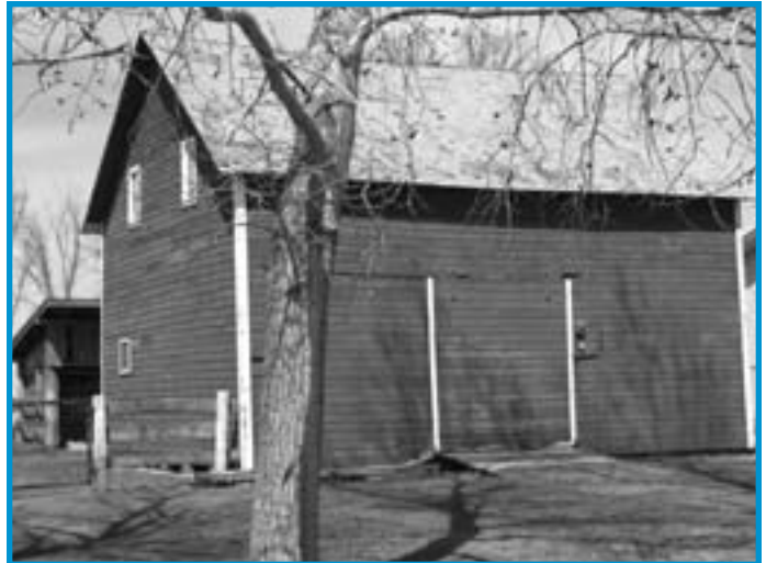
Granary roof is repaired
