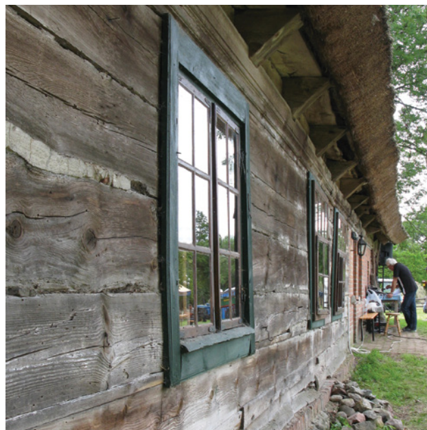
Exterior of Chrystowko House, 1770.
