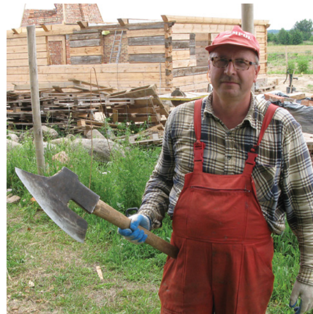
Reconstruction of Mennonite Housebarn in Torun.
