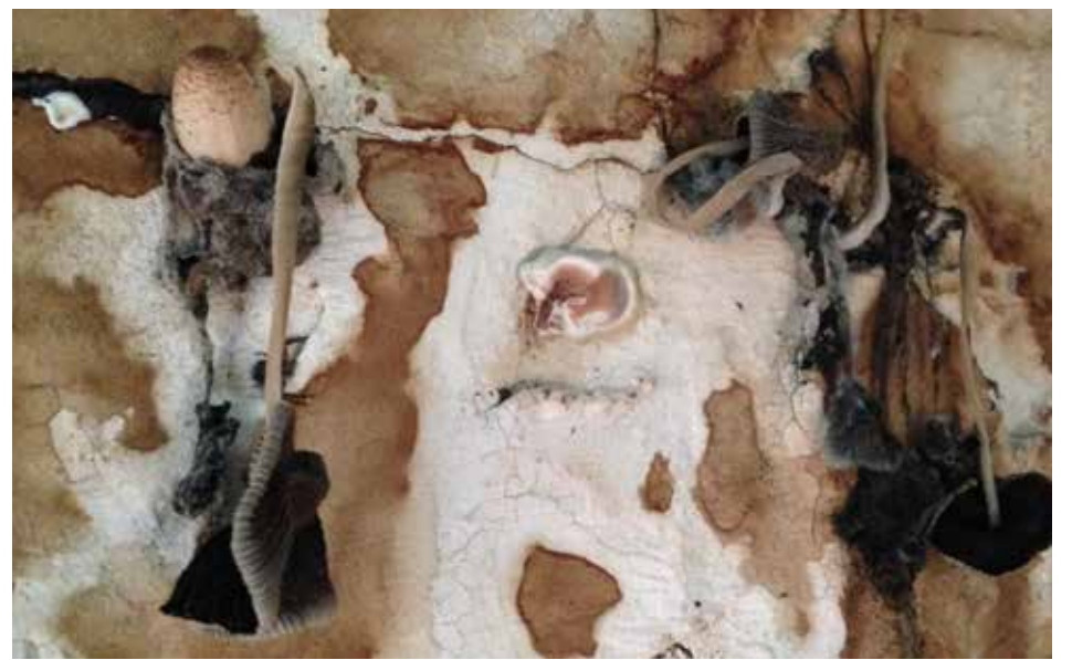
Example of fungi on the interior walls. Picture taken in September 2014.
