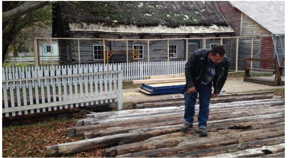
Jared Nickel, MHV's Facility Manager, inspecting the "new" oak logs, sourced from an 1890s log house in Sperling, Manitoba, that would replace the Waldheim House's rotten ones.
