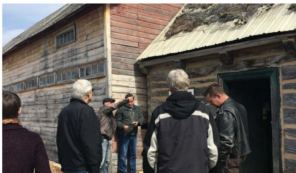
Discussing the upcoming roof thatching. (l-r) Alexandra Kroeger, Assistant Curator; Lloyd Dueck, volunteer; Myron Hiebert, Walls that Speak; Colin McGhee, McGhee & Co.; Barry Dyck, MHV Executive Director; Jared Nickel, Facility Manager
