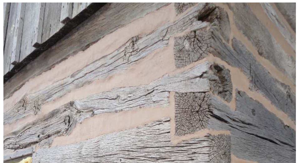
New chinking will provide much-needed protection from the elements.
