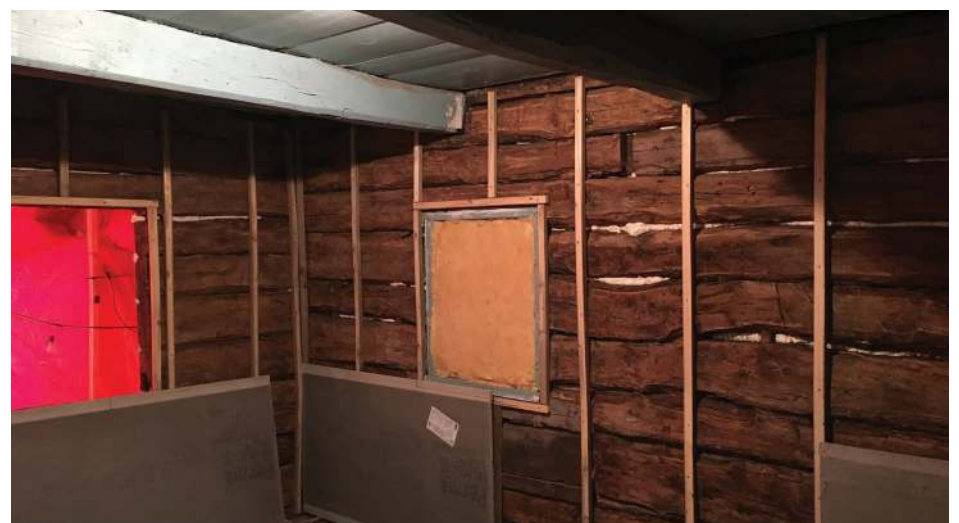
Interior walls being prepped for the new cement wall board.
