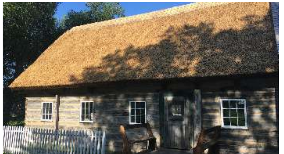
The Waldheim House, before and after. What a difference!
