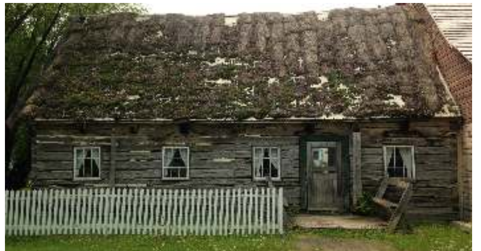
The west side of the house. Notice how thick the layer of reeds is.
